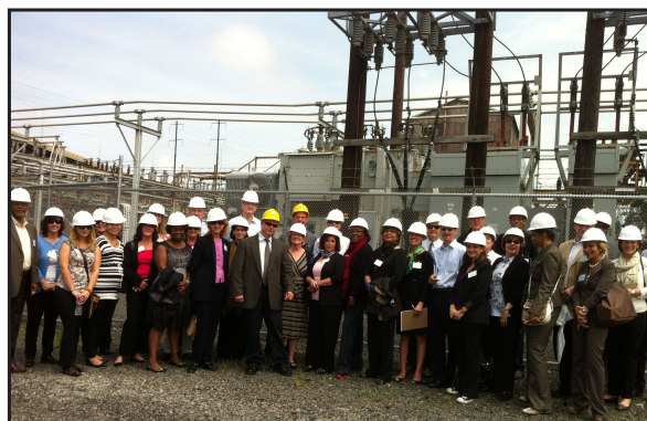
CNJG members toured the PSEG substation in Newark at the post-Sandy Site Visit to Urban Communities Affected.
